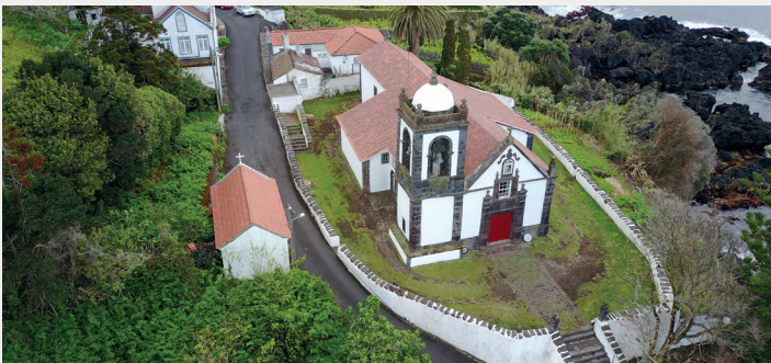
Aerial view of Manadas Church.
